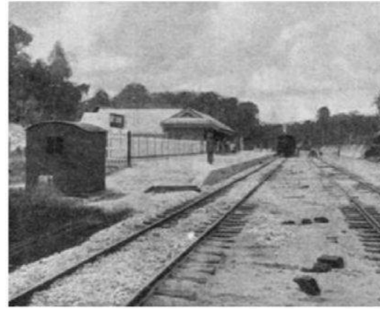
First coal release from the Kuang-Batu Arang (KTM) railroad construction.
