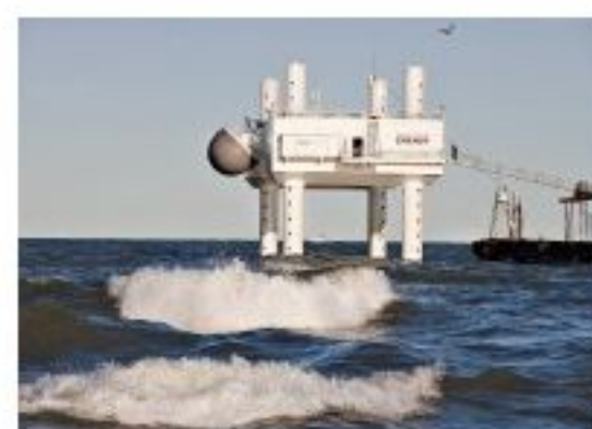
General view of Wave Star Energy's new 500-kilowatt test section located at the North Sea outside Hanstholm, Denmark. The floats produces energy by being lowered down to the surface of the sea and moved by the waves. Picture: EPA
